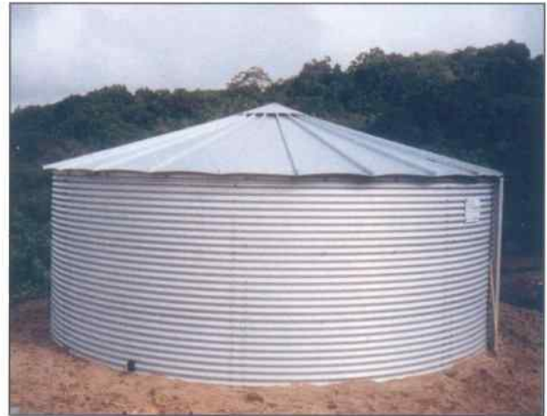
Illustration of Cone style roofed tank.
